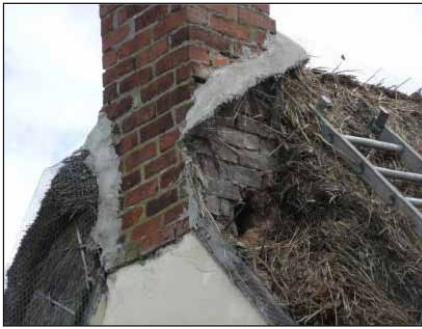
Figure 34. Thatch by imperfect chimney brickwork.
