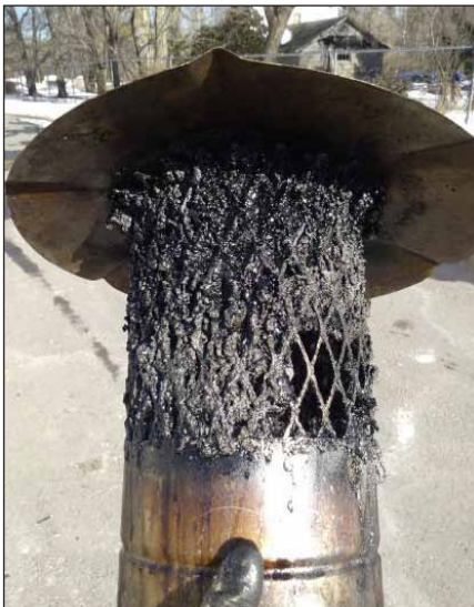
Figure 35. Tarred up chimney bird guard.
