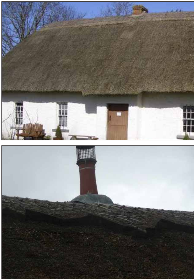
Figure 28. Thatched property with very small pot top to thatch clearance. Figure 29. Long-pot used to increase thatch to pot top clearance.
